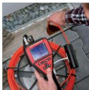
Inspection of rain drainage pipes
