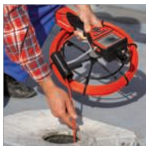
Inspection of rain downpipes
