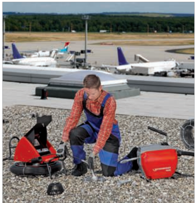
Inspection of a rainfall drains
